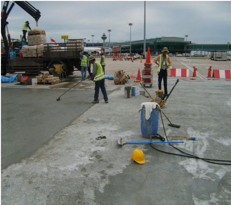
Semi-rigid Pavement for Airport Parking Aprons Construction in Progress 1 st time used in parking apron in Singapore
