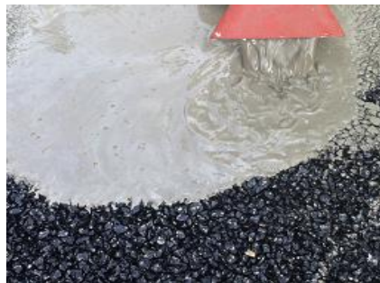
(b) Polymer Modified Cementitious Grouting Material filling into PAC
