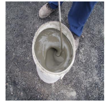
(c) Mixing With Hand Mixer (25kg powder/batch)
