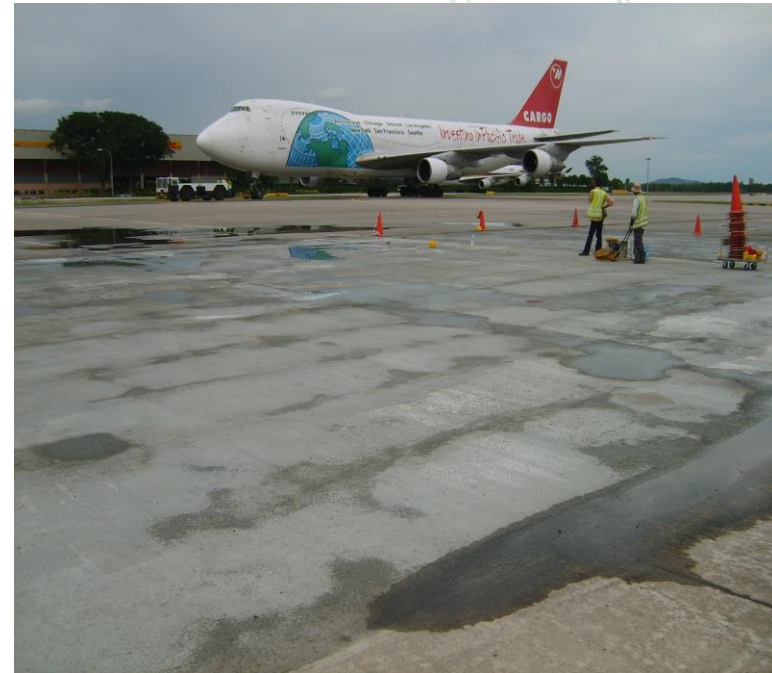
Semi-rigid Pavement for Airport Parking Aprons Construction in Progress 1 st time used in parking apron in Singapore
