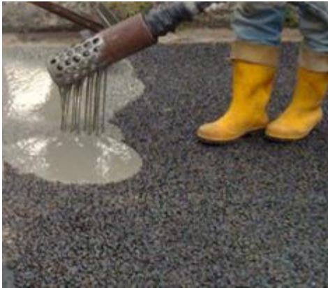
(a) Filling the grouting material into PAC
