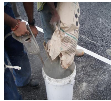
(c) Mixing With Hand Mixer (25kg powder/batch)
