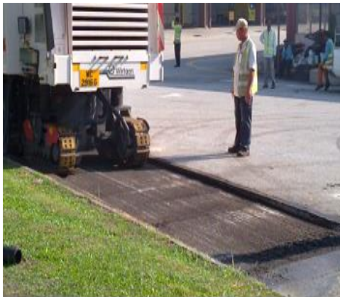
(a) Milling of Existing AC Surface
