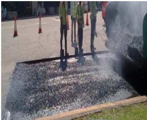
(d) Laying PAC to Designed Thickness
