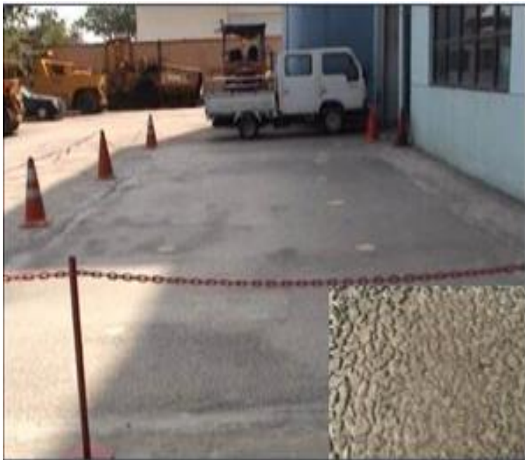
(a) Semi-Rigid Pavement after Hardened
